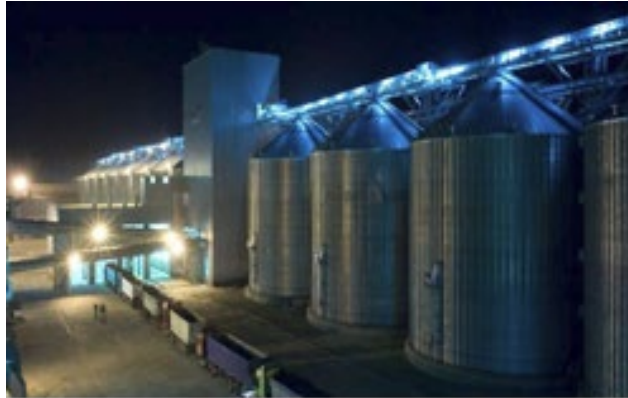
ADM Romania Logistics: EU project initiated in Constanta to increase grain handling capacity
